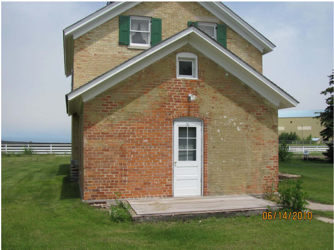
Figure III.6: Photograph of the current Ontonagon lighthouse structure. (Lisa Gillis, June 14, 2010.)
