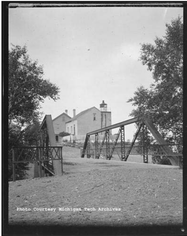
Figure II.15: Photograph of the second Eagle River lighthouse structure. (Michigan Technological University Digital Archives Image #MS-042-Z421, permission to reuse from MTU archives)
