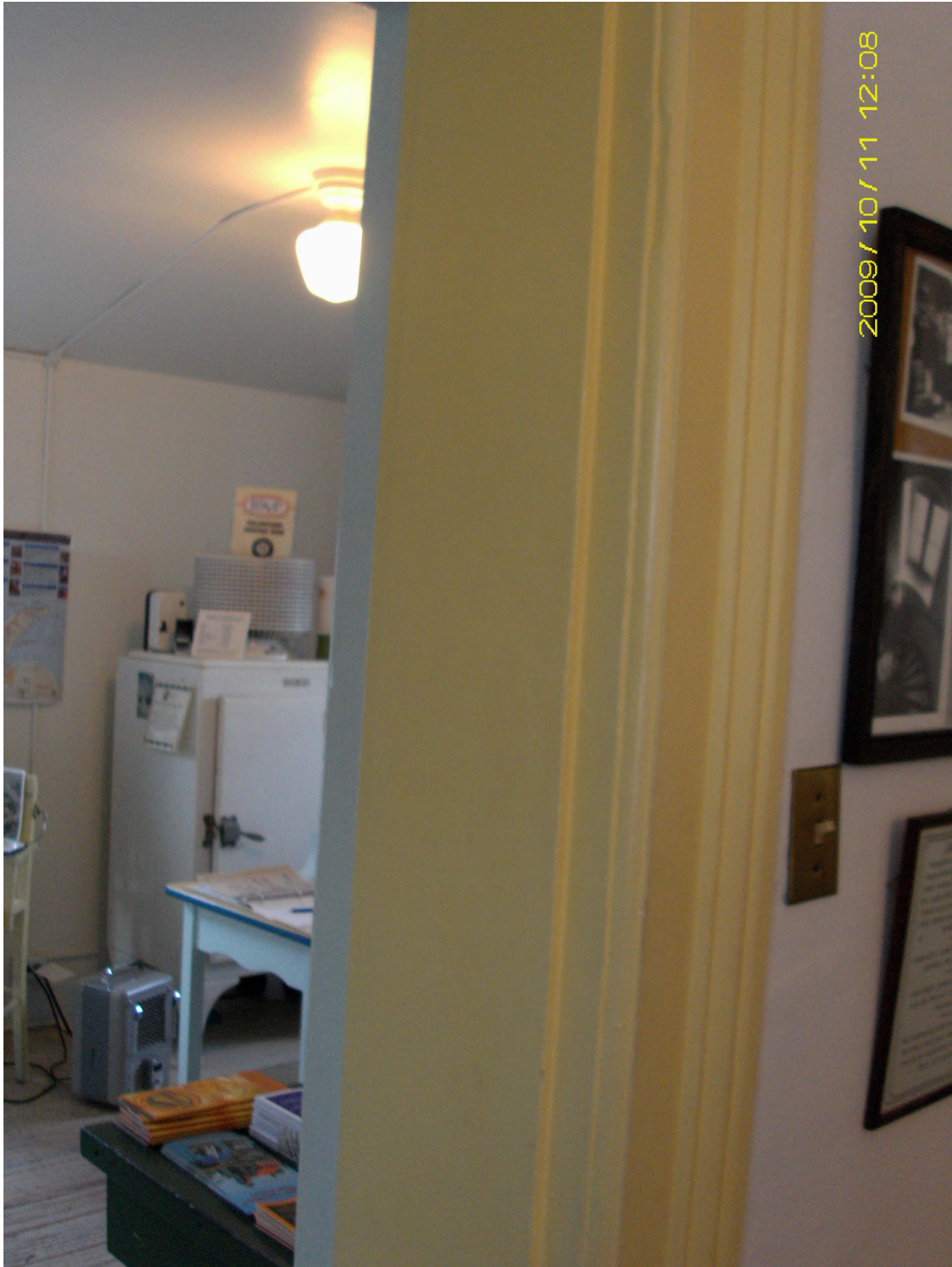
Figure III.5: Photograph of the wall thickness caused by poured concrete between two layers of brick. (Lisa Gillis, October 11, 2009.)
