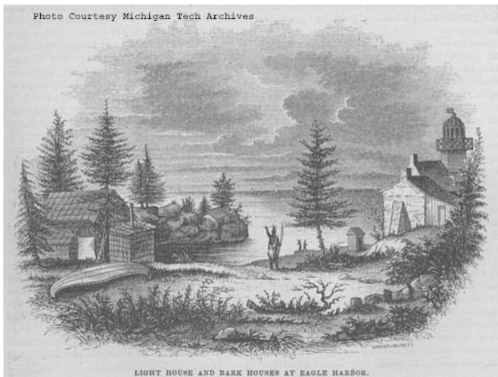
Figure II.11: Representation of the first Eagle Harbor lighthouse structure. (Michigan Technological University digarch #AP2H2v6-442-A, permission to reuse from MTU archives)
