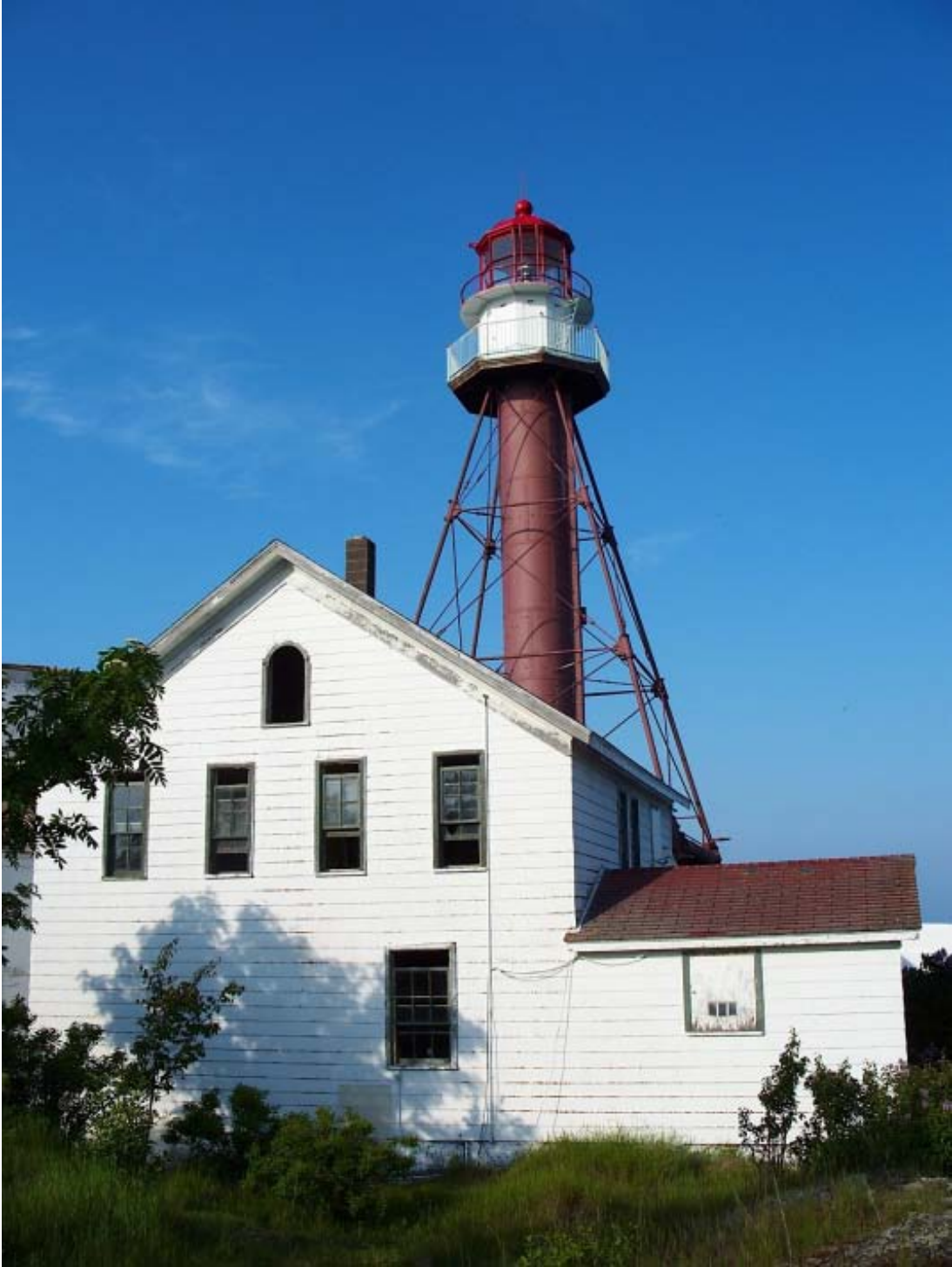
Figure III.3: Photograph of the current Manitou Island Lighthouse structure. (courtesy of the Keweenaw Land Trust, permission to use from Joe Kaplan)
