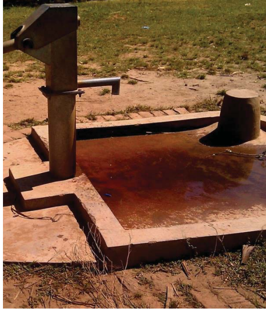
Figure 8: Iron-stained borehole
