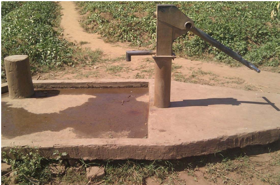
Figure 4: Borehole with Afridev hand pump
