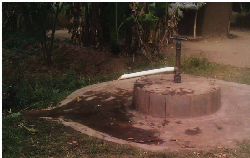
Figure 5: Shallow well with Mark V hand pump
