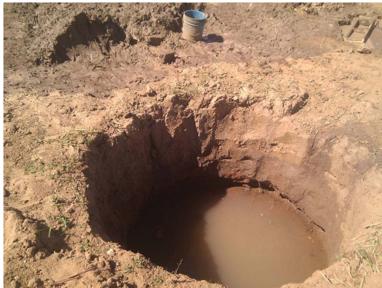
Figure 3: Water access pit dug for brick making
