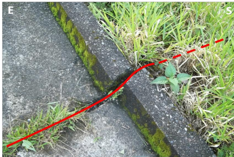
Fig. 20: deformation Chi4 and its length (top), particular of the indication for the lateral strike slip (bottom).
