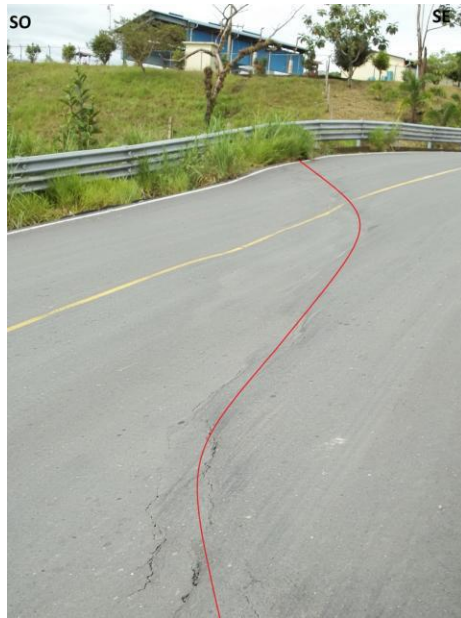
Fig.15: road deformation (HRev1) (photo by D. Alami).
