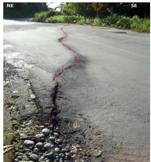
Fig. 16: Deformation of concrete slab along the road and length of the deformation(HRev2)(Photo By M. Balconi).
