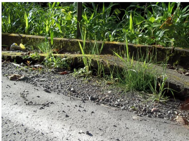
Fig. 16: Deformation of concrete slab along the road and length of the deformation(HRev2)(Photo By M. Balconi).
