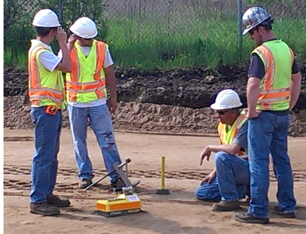
Figure 2.1 Troxler Nuclear Density Gauge (NDG)
