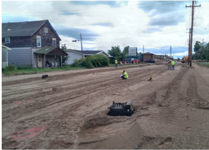
Figure 4.4 Subbase Sand Test Section at Iron River Site
