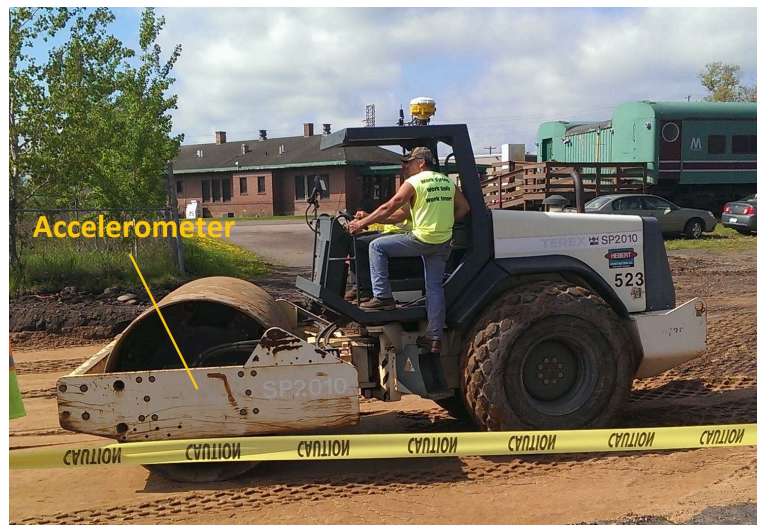
Figure 1.1 IC Unit Utilized in The M-189 Reconstruction Project
