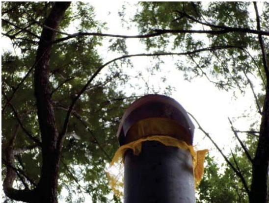
Figure 69: Completed ventilation tube with attached 'roof.' Photo by author.
