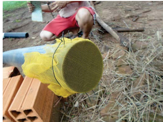
Figure 68: Attaching plastic screening to top of ventilation tube to prevent insects from entering. Photo by author.
