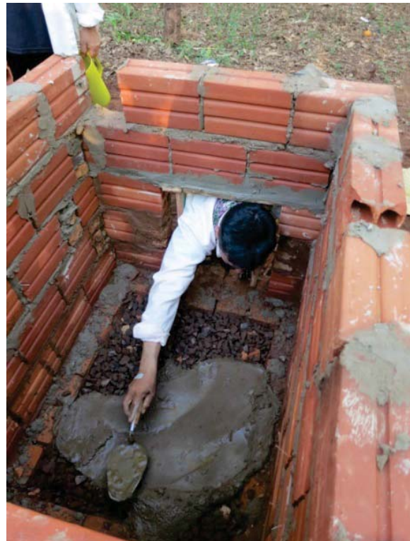
Figure 38: Vault floor being poured. Photo by author.
