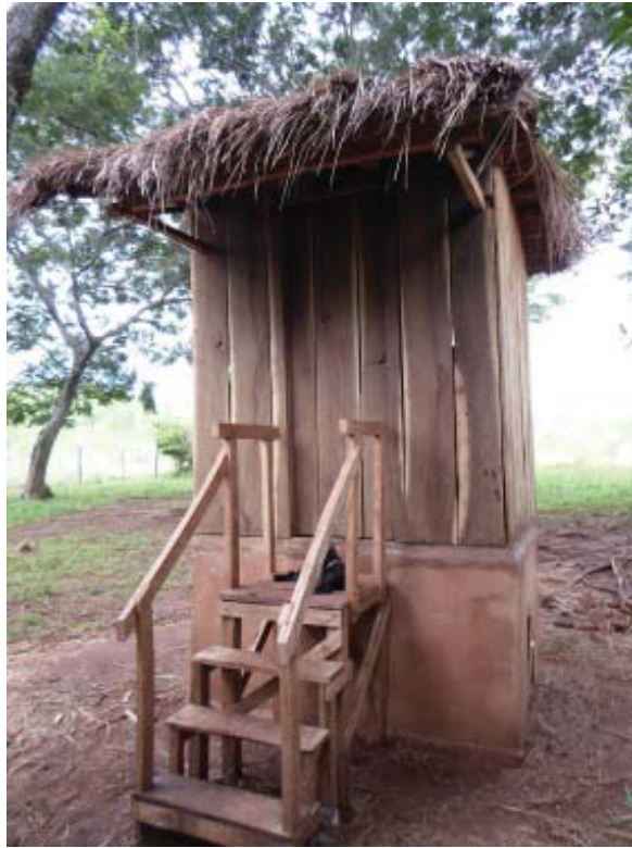
Figure 65: Author's completed latrine with thatch roof. Photo by author.
