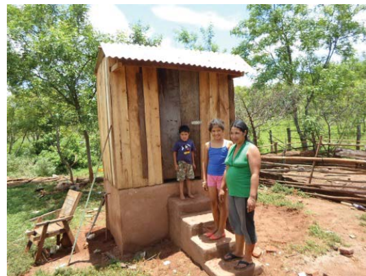
Figure 78: Finished four level brick steps. Photo by author.
