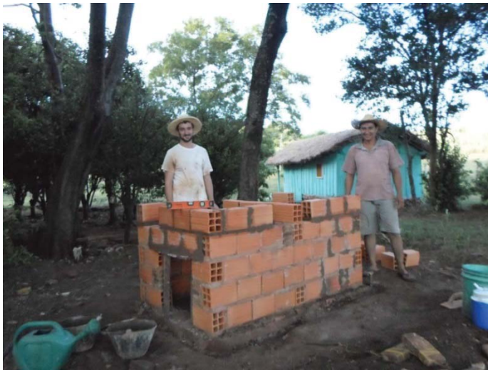
Figure 8: Author with his neighbor Io on completion of bottom of vaults of latrine. Photo by author.
