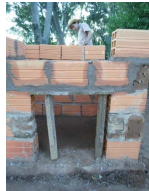
Figure 35: Completed 'bridge' over door opening. Photo by author.
