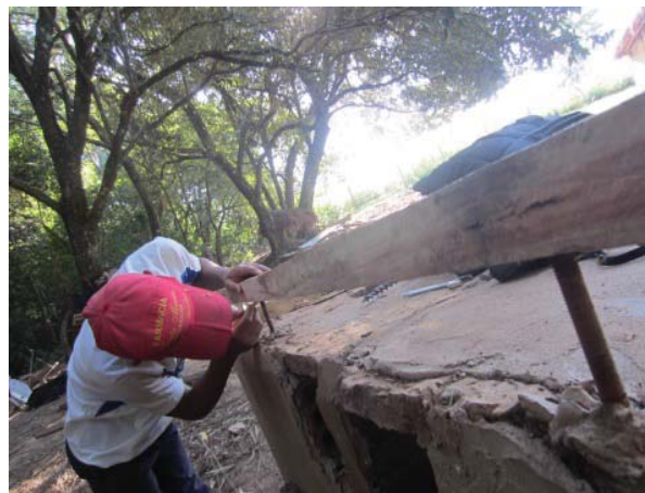
Figure 50: Lining up footer with threaded bars to prepare for drilling.
