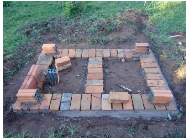
Figure 28: Corner bricks laid on first level. Photo by author.
