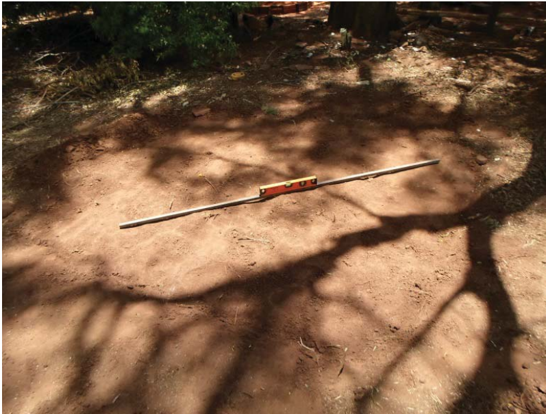
Figure 22: Level ground using shovel, hoe, rake, and long ruler. Photo by author.
