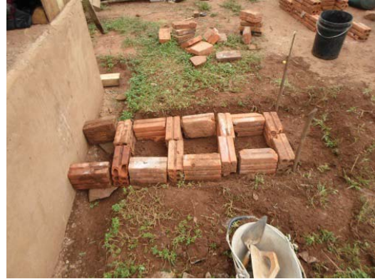
Figure 76: Base layer of brick steps. Photo by author.
