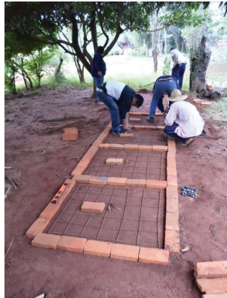
Figure 11: Tying rebar during loza construction. Photo by author.
