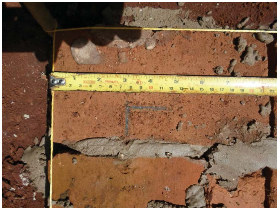
Figure 27: Corner brick placement marked 7.5cm from each side. Photo by author.
