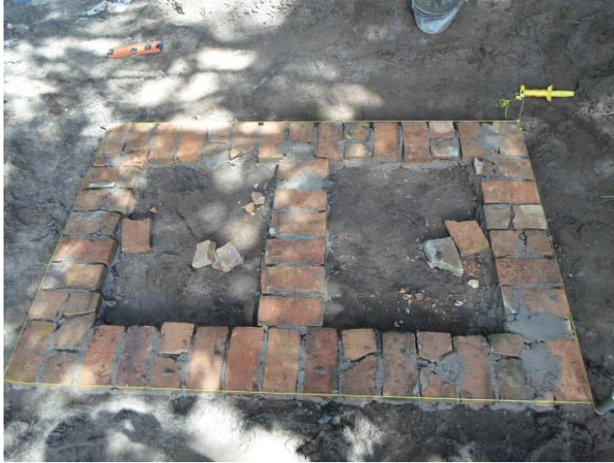
Figure 26: Completed base level of bricks. Photo by author.
