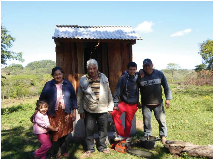
Figure 15: Completion day of this family's latrine. This latrine was built without help from the author. Photo by author.
