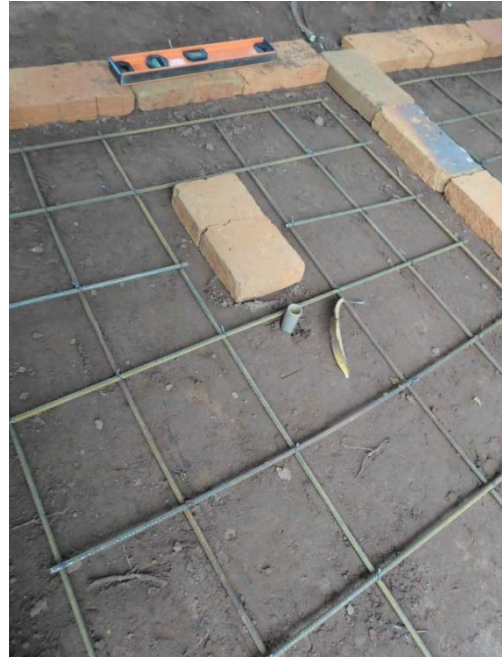
Figure 19: Placement of 20mm tubing in relation to loza opening. Photo by author.
