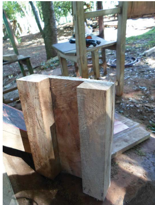
Figure 83: Back view of plastic covered board with post. Photo by author.
