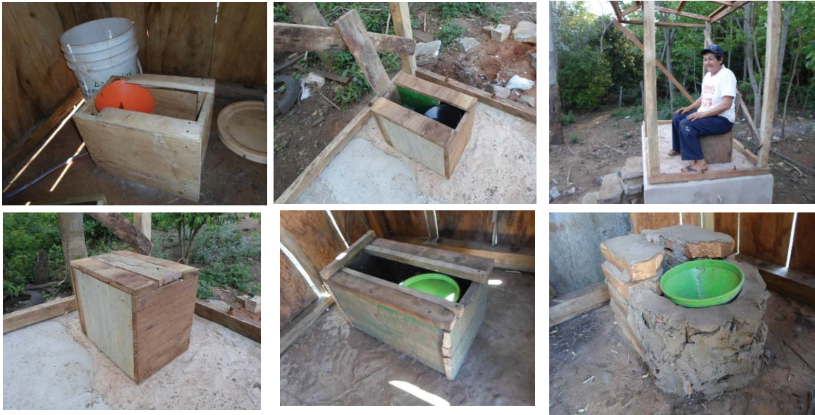
Figure 79: Six different urine diverting seats. Photos by author.
