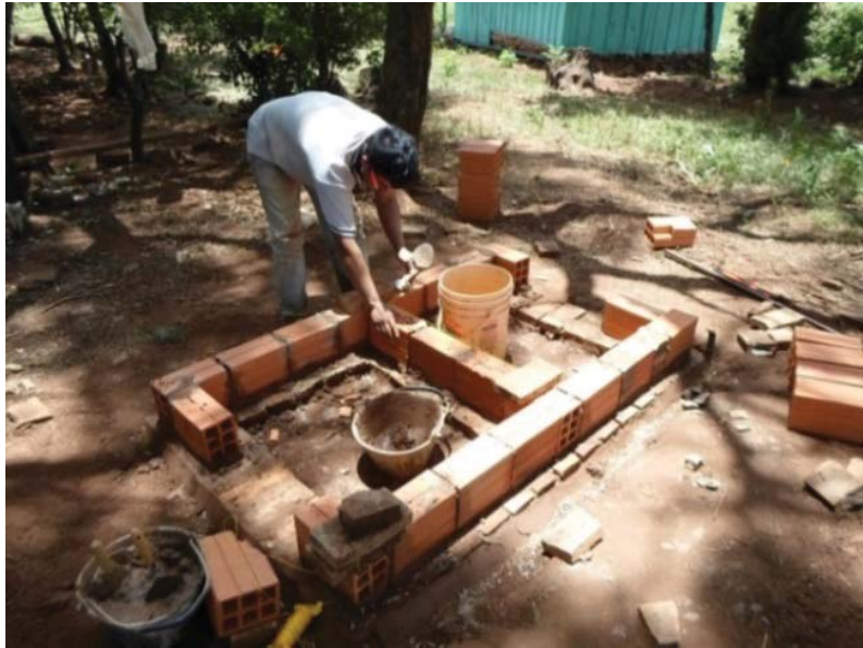
Figure 30: Center bricks of bottom layer being laid. Photo by author.
