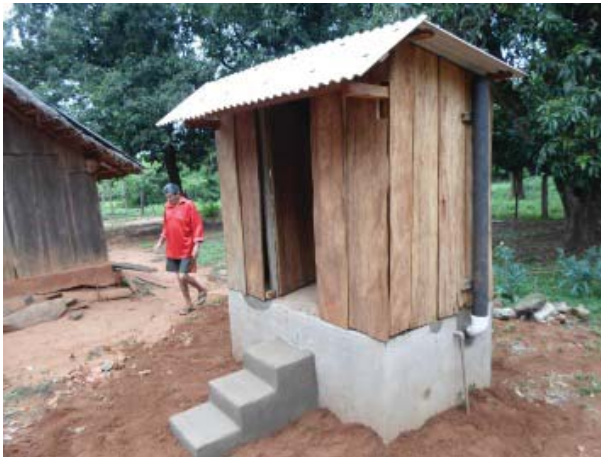
Figure 77: Finished three level brick steps. Photo by author.
