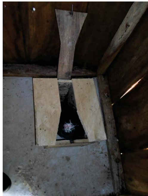
Figure 90: Completed seat with plastic burlap 'strainer' placed in funnel. Photo by author.
