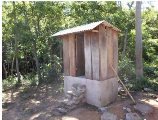
Figure 64: Completed latrine with chapa roofing material. Photo by author.
