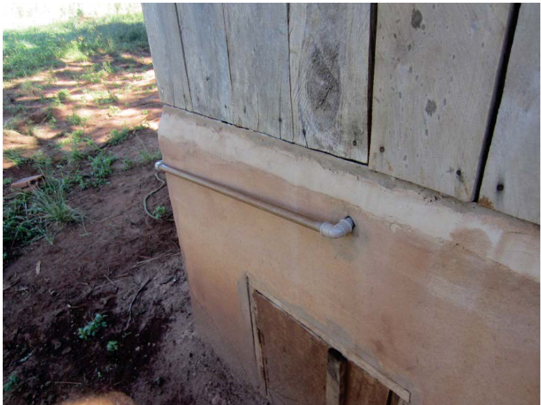
Figure 92: Placement of 20mm PVC urine diversion pipe. Photo by author.
