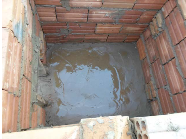
Figure 39: Completed floor of vault. Photo by author.
