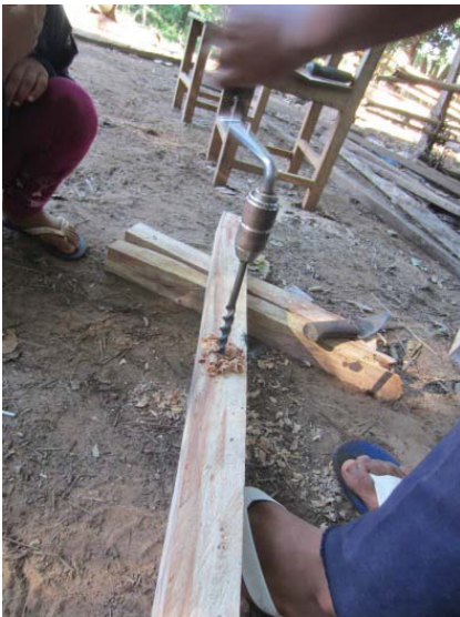
Figure 53: Drilling footer with 5/8" bit. Photo by author.
