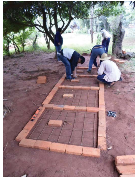
Figure 16: Tying of rebar during loza construction. Photo by author.
