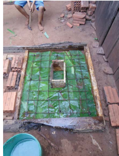
Figure 17: Completed rebar cage. Photo by author.
