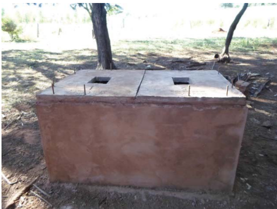
Figure 49: Completed base of latrine. Photo by author.
