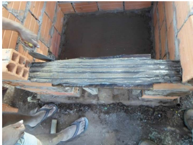
Figure 34: Placement of mortar in-between and below rebar. Photo by author.
