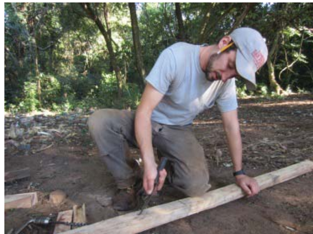
Figure 54: Cleaning drilled holes with knife. Photo by author.
