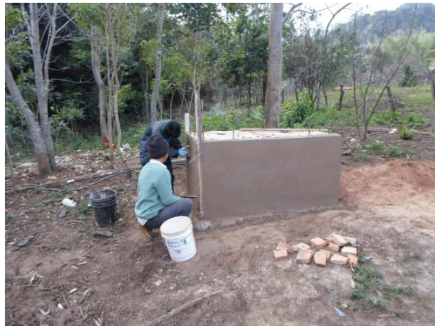
Figure 48: Final smoothing of latrine outside walls. Photo by author.
