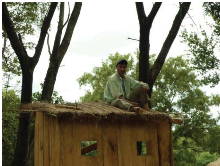
Figure 66: Completing roof with thatch. Photo by author.
