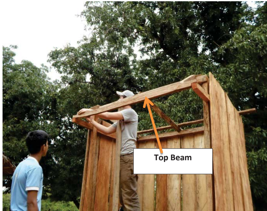
Figure 59: Top beam placement. Photo by author.
