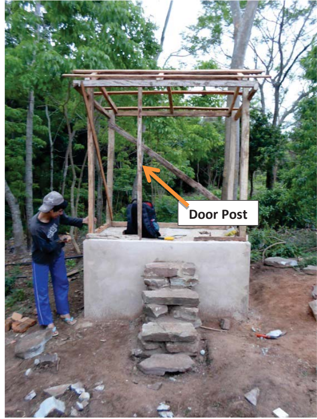
Figure 60: Door post placement. Photo by author.
