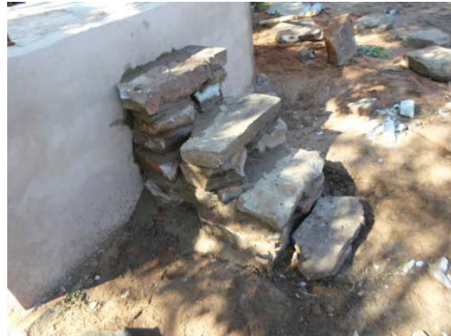
Figure 74: Completed rock steps. Photo by author.
