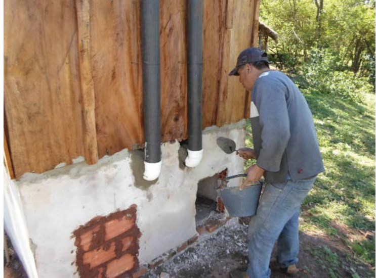
Figure 70: Attaching ventilation tubes to housing structure. Photo by author.
