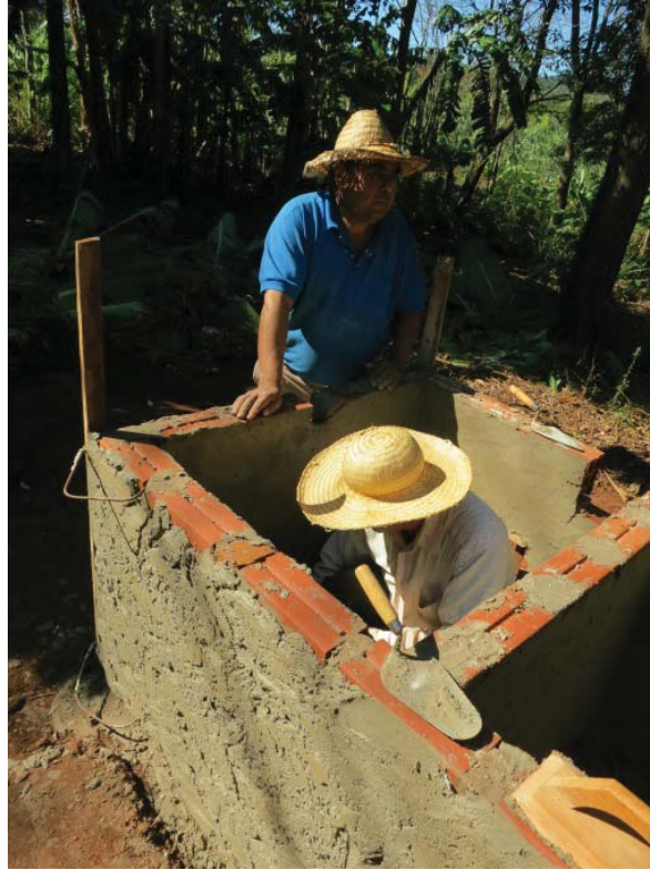
Figure 12: Construction of first commission latrine. Photo by author.
