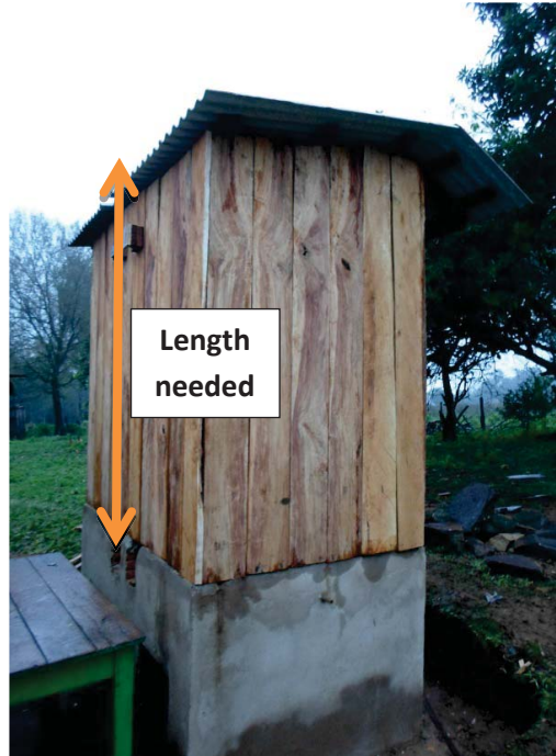
Figure 67: Length of tubing needed measured from opening to 10cm above roof. Photo by author.
