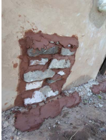
Figure 95: Vault closed with rocks and clay mortar. Photo by author.
