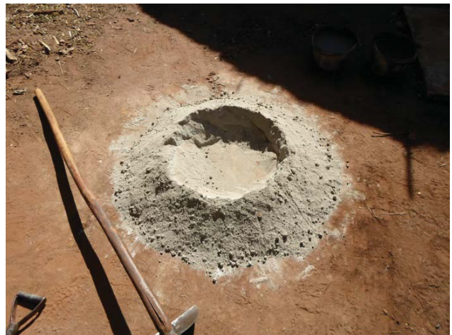
Figure 23: "Volcano" method of mixing concrete. Photo by author.
