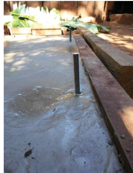
Figure 20: Threaded bolts placed 5cm from edge of loza . Photo by author.
