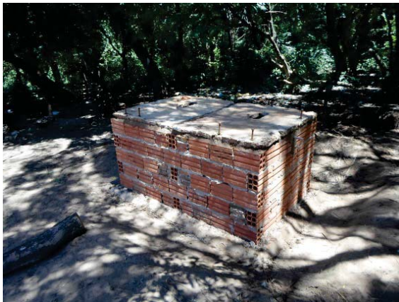
Figure 44: Completed latrine base without stucco on outside walls. Photo by author.
