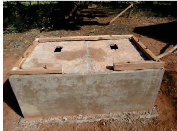
Figure 56: Completed footer installation. Photo by author.
