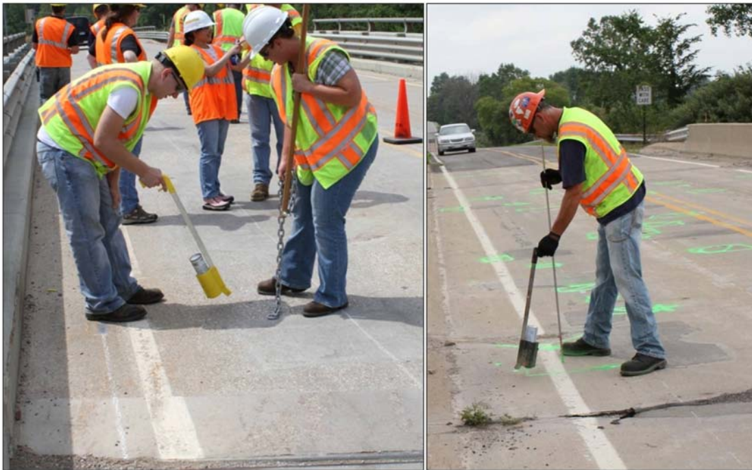
Figure 2.2 Chain drag and hammer sound techniques.
