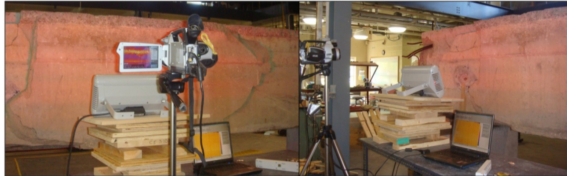
Figure C.6 Active infrared thermography test set-up at the location E3.
