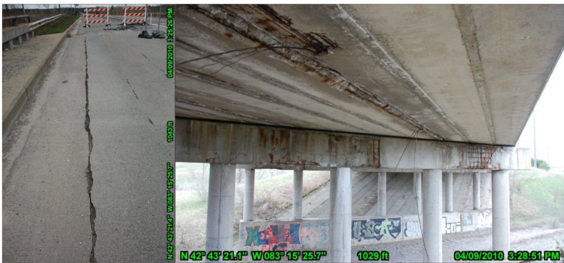
Figure 6.5 Silverbell Bridge deck and superstructure in April 2010.
