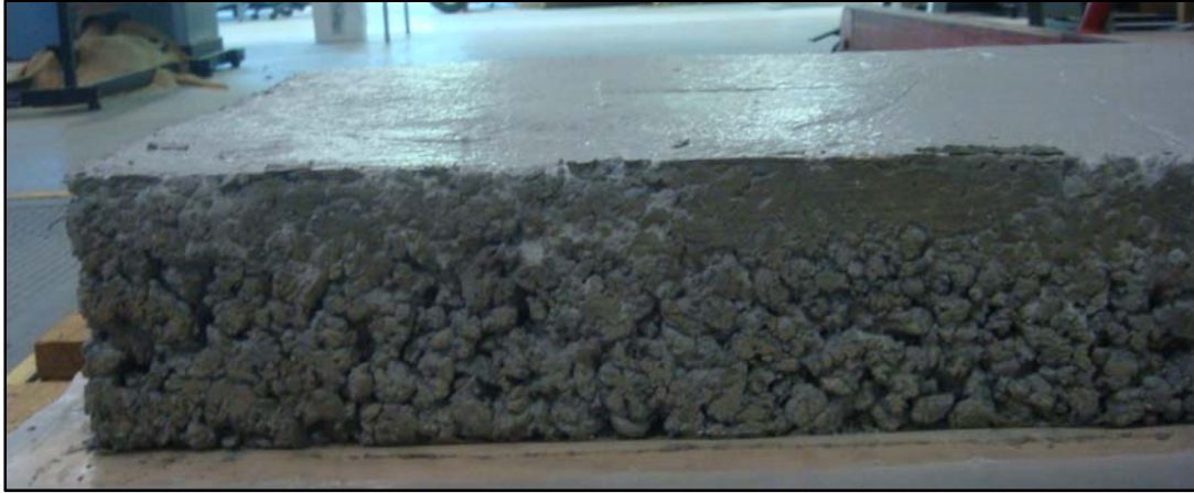
Figure 5.37 Slab II after the timber form was removed.
