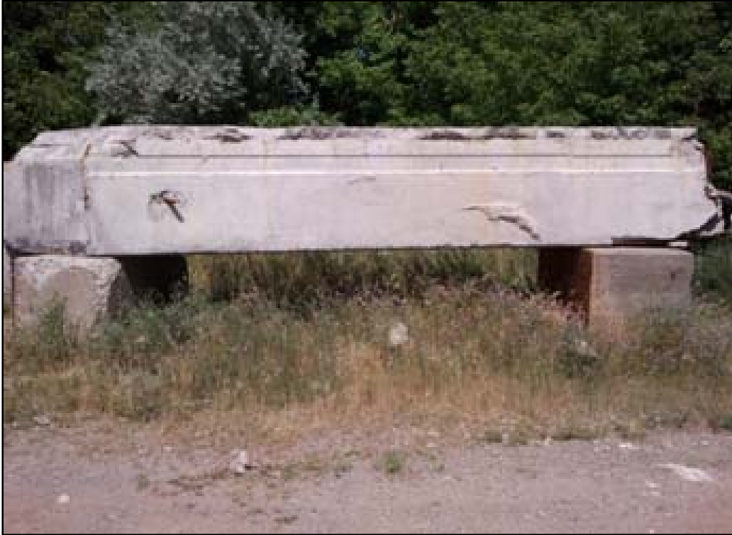
Figure 6.6 Silverbell Bridge beam in Road Commission Oakland County facility (west face shown).
