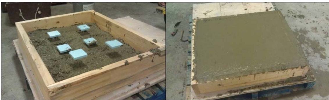
Figure 5.2 Construction sequence of the concrete slab with Styrofoam blocks used as simulated delaminations.
