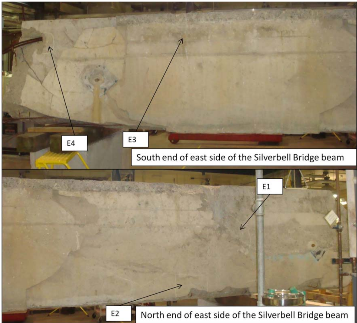
Figure 6.9 East side of the Silverbell Bridge beam.
