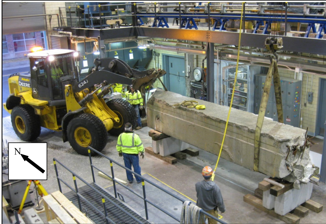
Figure 6.7 Placement of Silverbell Bridge in the Michigan Tech laboratory.
