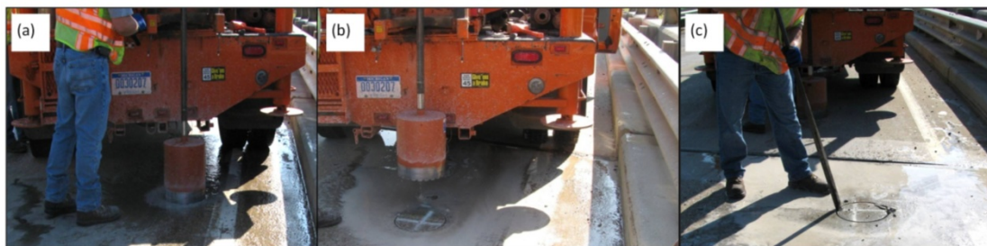
Figure 4.18 Core extraction procedure on Mannsiding Rd. bridge deck.
