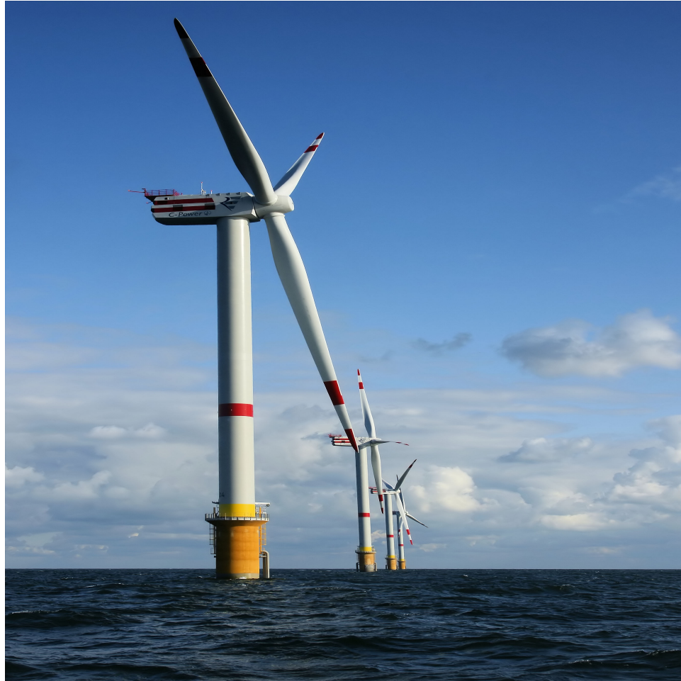
Figure 1.1: The REpower M5 5-megawatt turbine, with a rotor diameter of approximately 126 meters (from (5)). Permission to reuse in Appendix.
