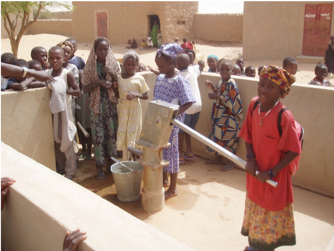
Figure 6: Photograph of the India Mark II hand pump (image courtesy of Michael MacCarthy)
