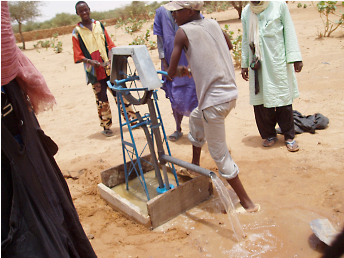
Figure 5: Photo of a rope pump installation, apron not shown (image courtesy of Michael MacCarthy)
