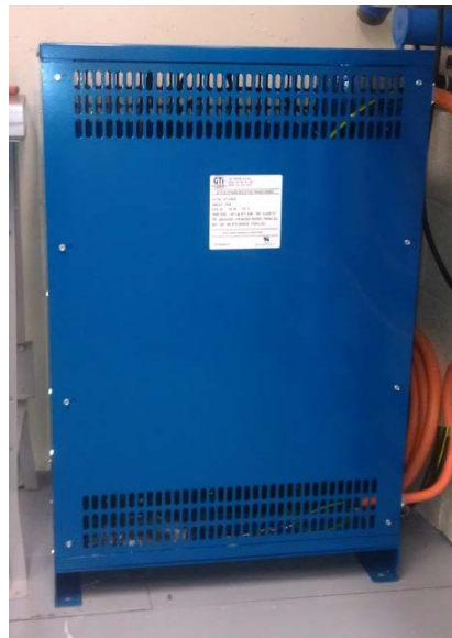
Figure 3.4: Isolation Transformer
