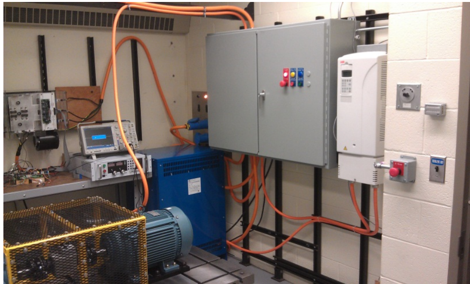
Figure 2.10: Completed Test Cell System
