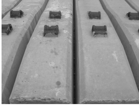
Figure 6: Non-captive PANDROL E-CLIP fastening system
