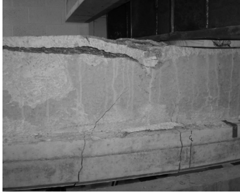
Figure 31: Prestressed concrete beam failure corresponding to Figure 30, showing flexural cracking and crushing of the compression zone
