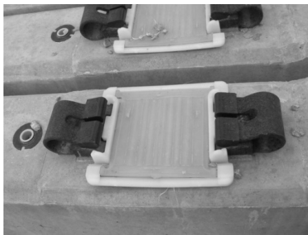
Figure 7: Captive PANDROL SAFELOK III fastening system
