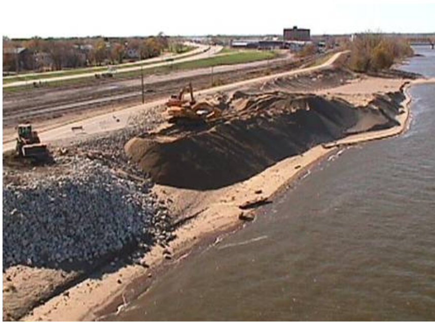
Figure 2.2: Fill/Construction Materials, Pool 16 UMR
