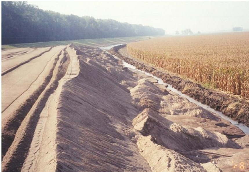
Figure 1.9: Behind Levee Placement
