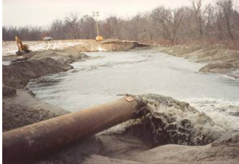
Figure 1.6: Cutterhead Pipeline Dredge Discharge
