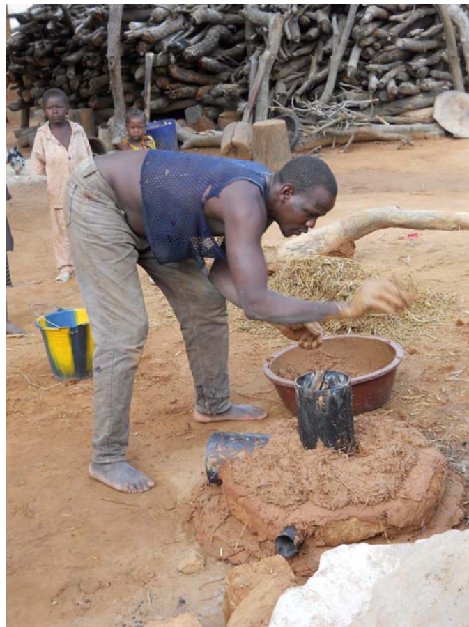
Figure 1-3 Stove construction in Mali (photo by author)
