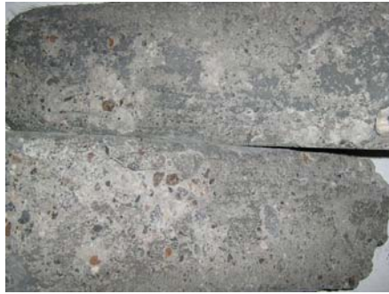
(a) B(C): Bond due to concrete failure.
