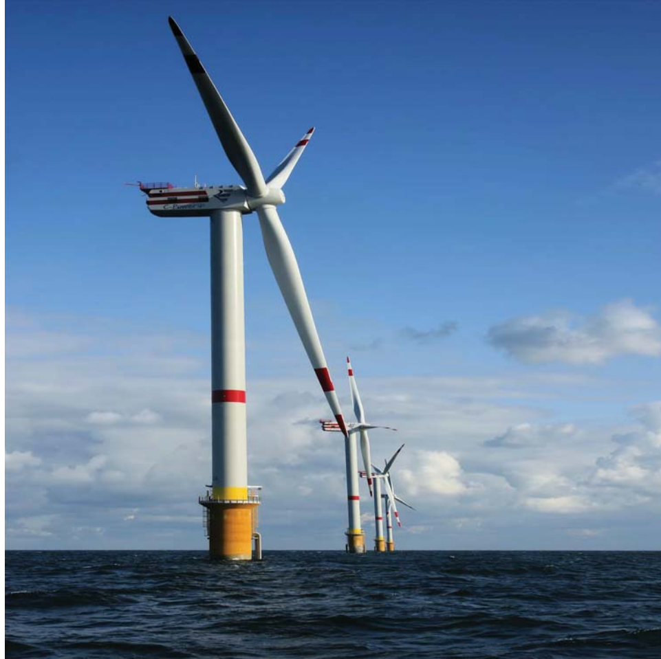
Figure 1.1: The REpower M5 5-megawatt turbine, with a rotor diameter of approximately 126 meters (from (5)). Permission to reuse in Appendix C.
