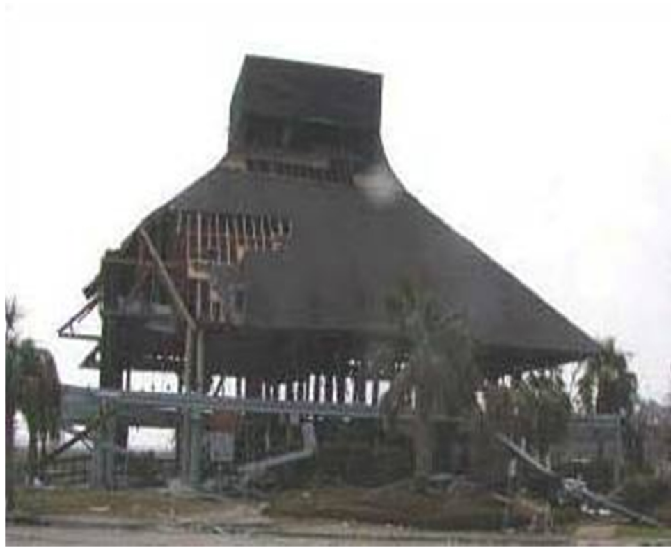
Figure 2.1: Wind and Storm Surge Damage
