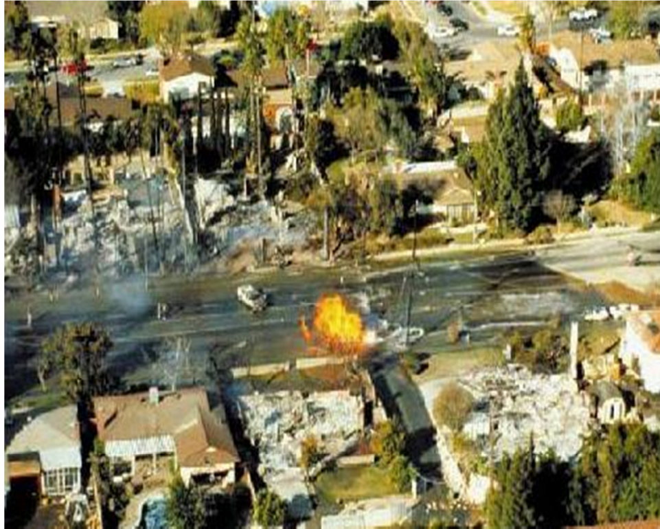
Figure 2.2: Fire from Damage to Gas Pipelines from Northridge Earthquake in 1994
