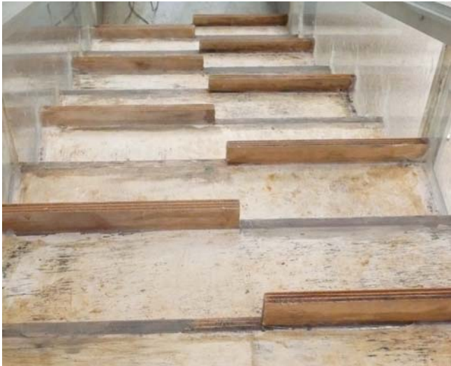
(D) Stepped spillway with staggered configuration of flat and pooled steps
