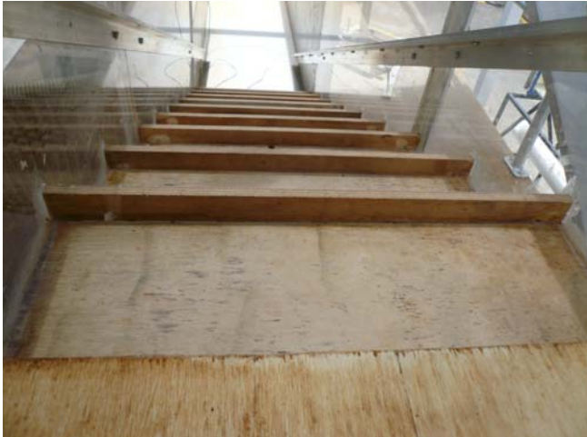
(B) Pooled stepped spillway
