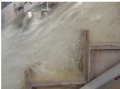
(B1) Visible flow resistance close to pool weir
