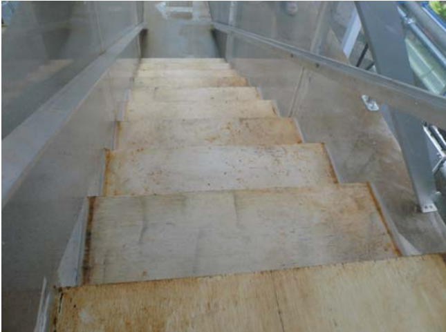
(A) Flat stepped spillway
