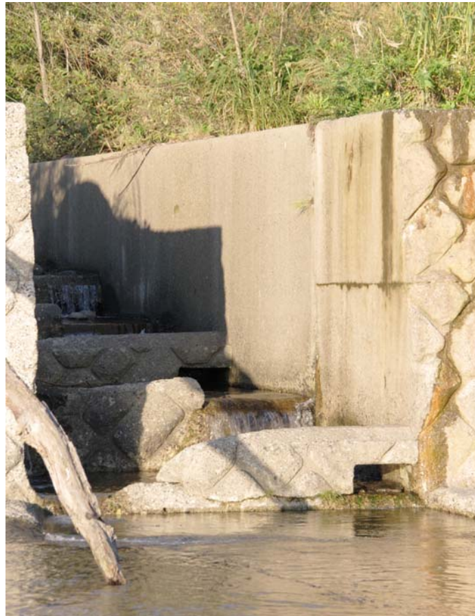
(B) Looking at the downstream end of a fully-silted fishway - Note the eroded step edges
