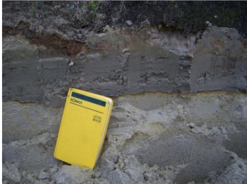
Figure 27: Favorable sediment conditions for the formation of liquefaction features at the Suncook River Avulsion site. For scale, the notebook is 19.5 cm tall and 11.5 cm wide.
