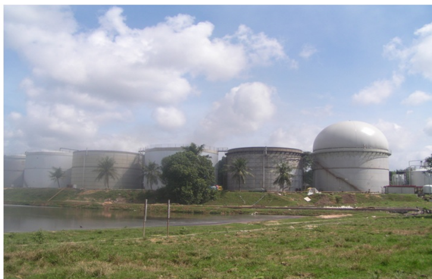
Fig. 3: The commercialization stage of the methane recovery project from anaerobic treatment of palm oil mill effluent in Seriting Hilir Palm Oil Mill, Negeri Sembilan, Malaysia.
