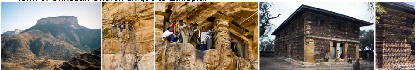
Debre Damo Monastery, The oldest surviving church in Ethiopia, founded in the 6 th Century, is located on a spectacular and remote mountain-top West of Adigrat. It is accessible only by rope. The exterior walls are constructed with alternating courses of limestone blocks and timber bands held together at right angles to the faces of the wall by cross timbers that project prominently on the exterior. These 'Monkey Heads' are a distinctive characteristic of Axumite architecture and can be seen celebrated in stone on the more elaborate Stelae in Axum. This building is the only genuine survivor of this style of building. The interiors of the church have many ancient original paintings.
