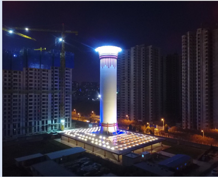
Figure B A night-view of the 1 st generation SALSCS built in Xi'an, Shaanxi Province (completed July 2016)
