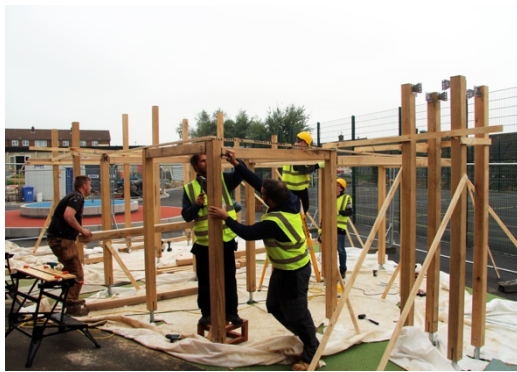
Playscape Construction. Image: PO
