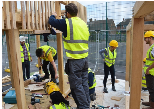
Playscape Construction. Image: PO
