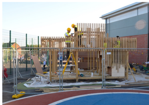
Playscape Construction. Image: PO
