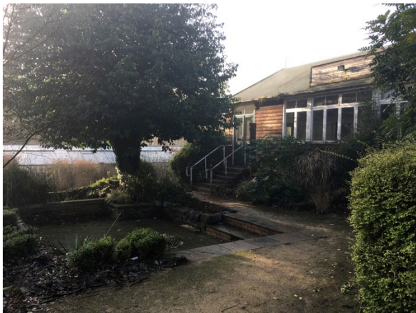
Existing LRC Building. Photo by PO
