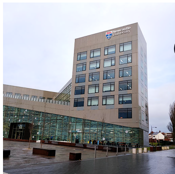
Figure 2: The Urban Sciences Building at Newcastle University. A Living Lab building designed to the BREEAM Excellent standard.
