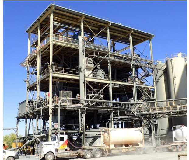
Figure 4. A typical open-framed mine process structure.
