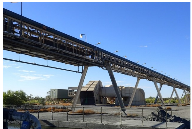
Figure 5. A typical mine elevated conveyor structure.
