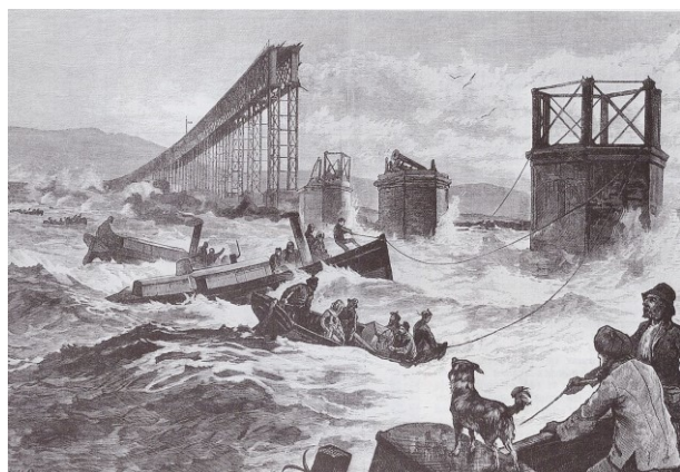
Figure 1. Tay Rail Bridge Disaster ( https://www.railwaysarchive.co.uk )
