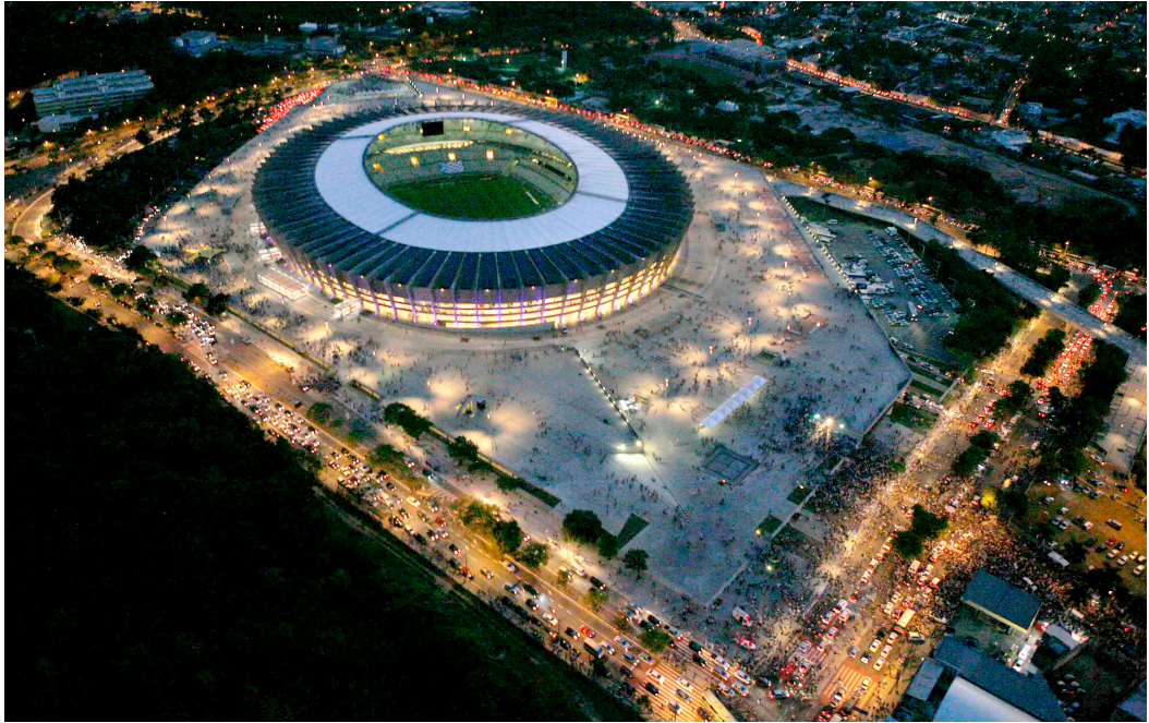
Figure 4.9. New Mineirão stadium
