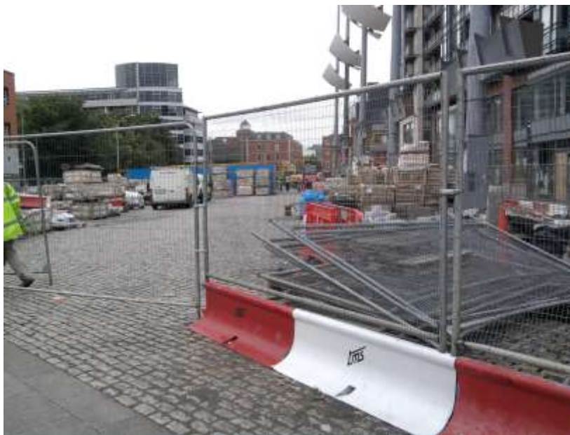
Figure 6 Still under construction 18th July 2011
