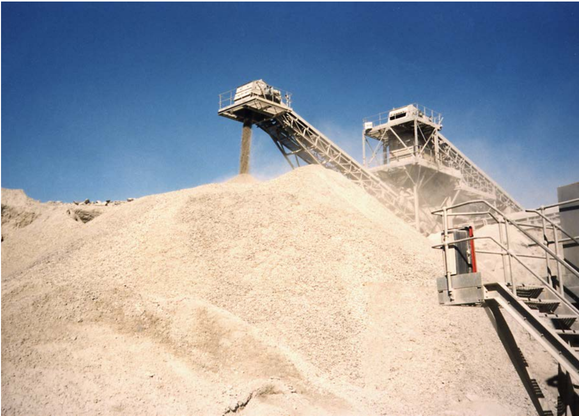
Coarse aggregate from the primary crusher, Leahill Quarry
