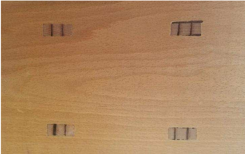
Fig.7. Tenon and mortise in the FLOS top plate surface
