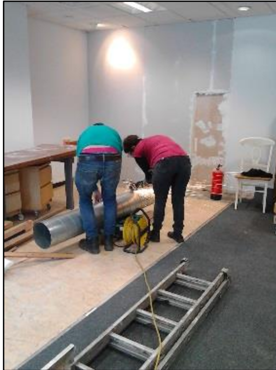
Figure 43: Remakery Under Construction I
