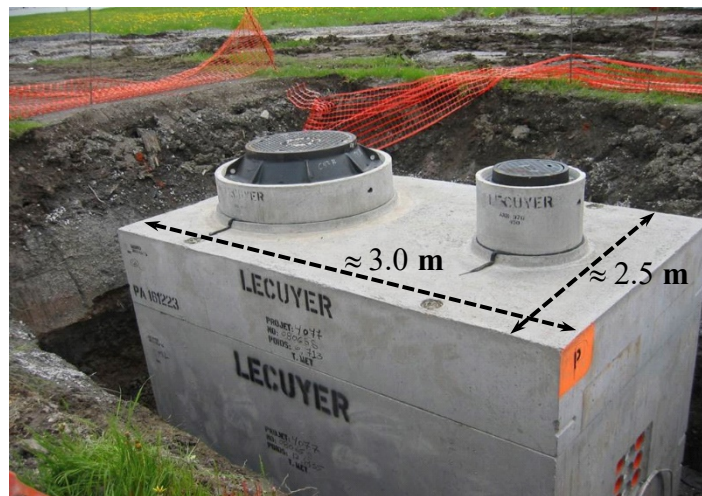
Figure 5.1 Typical underground utility structure.
