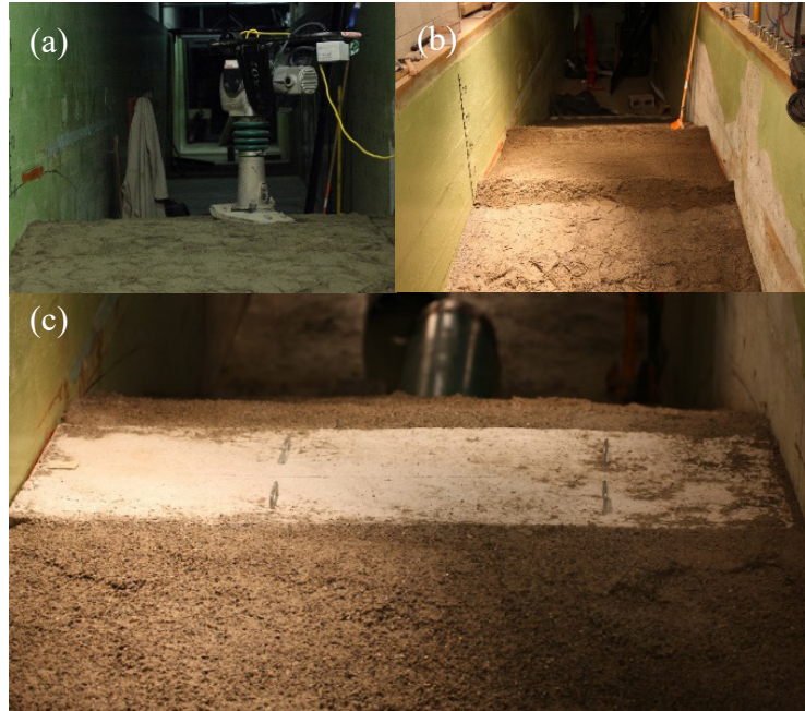
Figure 6.5 a) Placement and compaction of the soil; b) Experimental model E1; c) Experimental model E2 with the 0.06 m thick concrete slab on top of the model.
