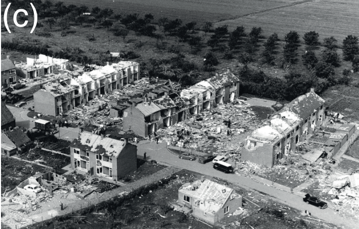
770 FIG. 3. Tornado damages associated with the (a) Pommereuil, (b) Palluel tornadoes from 24 June 1967 over 771 France (courtesy of Jean Dessens), and (c) Tricht tornado (Netherlands) from 25 June 1967 (courtesy of ANP 772 Historisch Archief).
