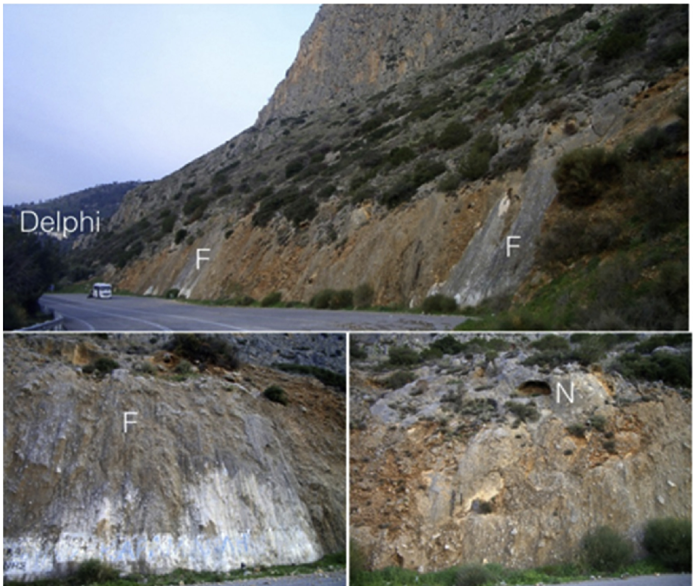
Fig. 8. (a) View looking west toward the the principal fault plane (F) at Delphi. (b) A close up of the fault plane (F) showing the polished and grooved surface, adorned enigmatic rock-cut niches (c).
