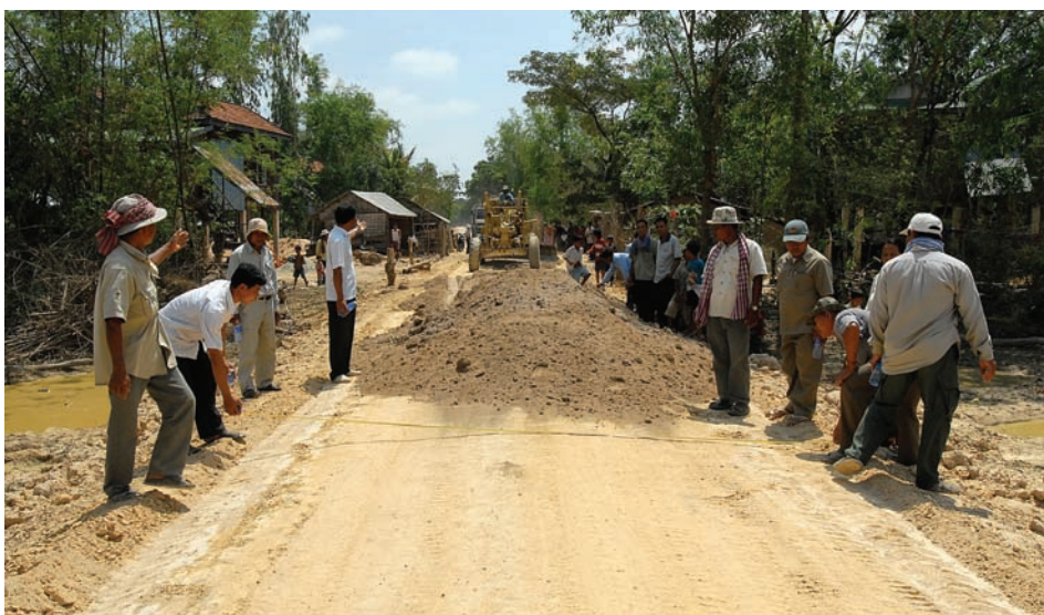
UNDP PHOTO Road construction in Cambodia.
