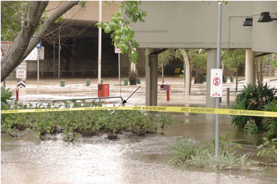
(B) Zoom into the boom gate pylon and the handrail supporting the ADV system (arrow)
