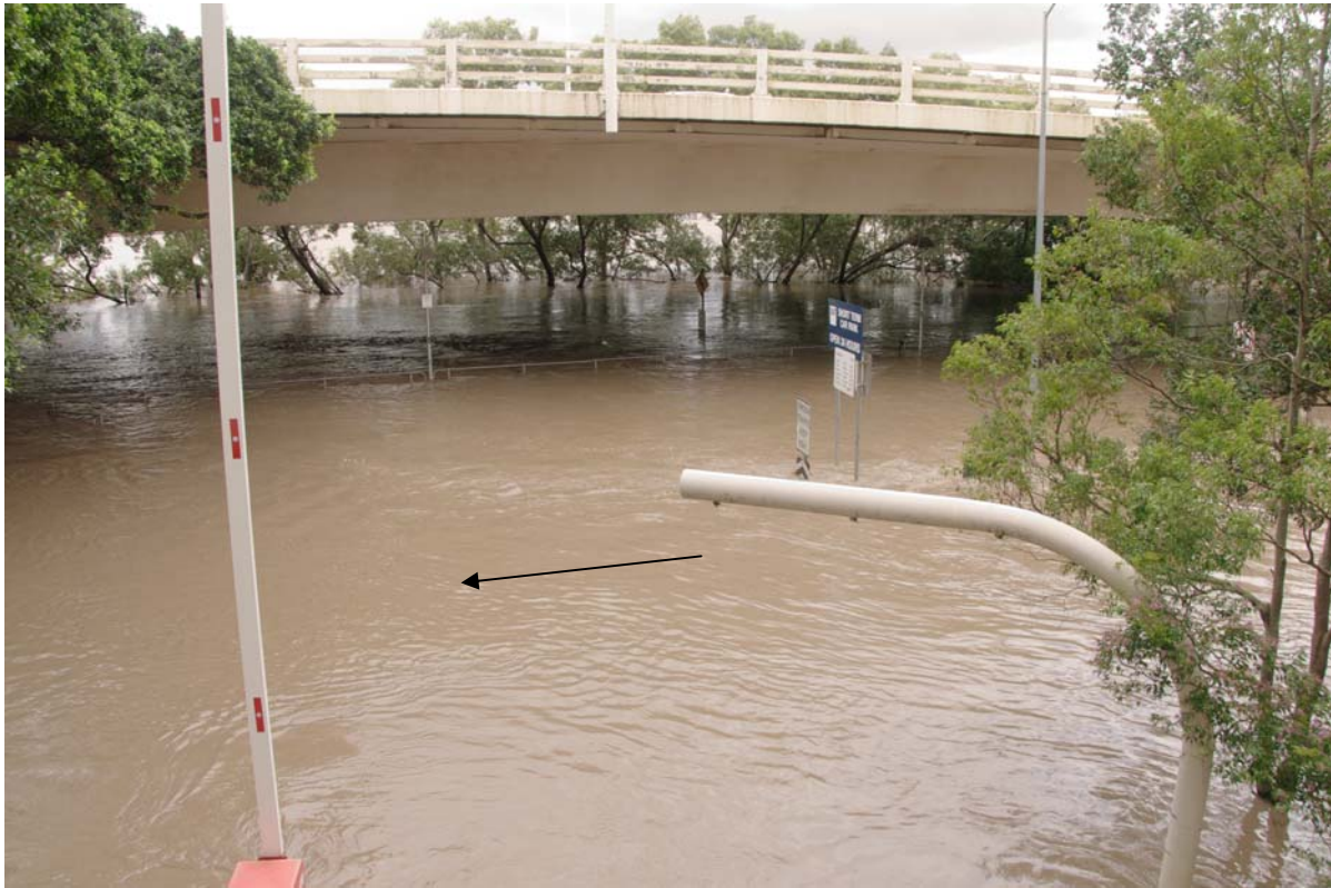
(A) General view of Gardens Point Road viewed from C Block parking level 2 on Thursday 13 January 2011 at 10:39 (Photograph Hubert CHANSON) - Flow from right to left, with Captain Cook Bridge in the background
