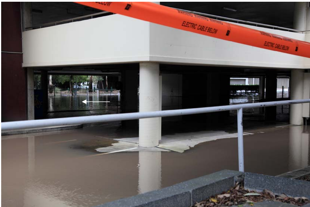
Fig. A-6 - Parking beneath C Block with Gardens Point Road in the background on Wednesday 12 Jan. 2011 at 10:18 (Photograph courtesy of QUT Facilities Management) - Canon™ 5D Mk II with Canon™ EF24-105mm F4L IS USM lens - Flow direction (arrow) from right to left
