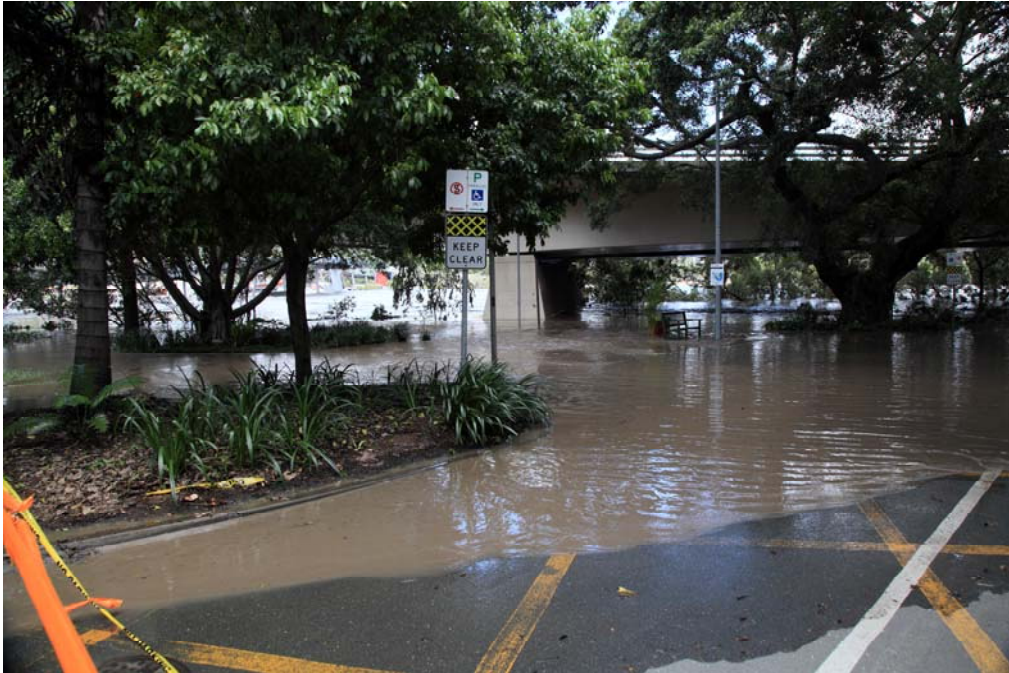
Fig. A-8 - Roundabout at the SE (downstream) end of Gardens Point Road on Wednesday 12 Jan. 2011 at 11:48 (Photograph courtesy of QUT Facilities Management) - Canon™ 5D Mk II with Canon™ EF24-105mm F4L IS USM lens - Flow direction from right to left
