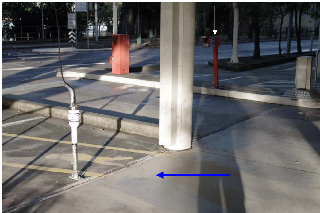
Fig. 2-7 - ADV on 14 January 2011 at 05:57 after the flood receded - The ADV unit is on the left while the boom gate pylon (white arrow) is seen in the right background, behind the concrete column - The blue arrow shows the main flow direction - Note that the parking concrete slab was
