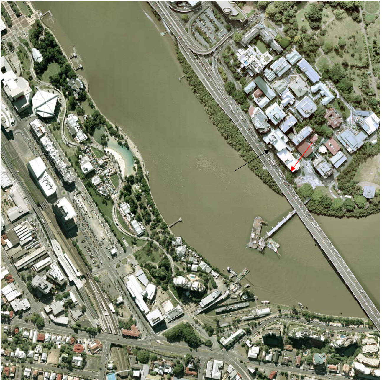
Fig. B-3 - Aerial photograph of Gardens Point during construction in 2001 (Copyrights QUT) - Brisbane River flow from top left to bottom right - The black arrow points to Gardens Point Road between Captain Cook Bridge and the C-Z-S Blocks, while the red arrow points to the ADV location - Note the Goodwill Bridge under construction
