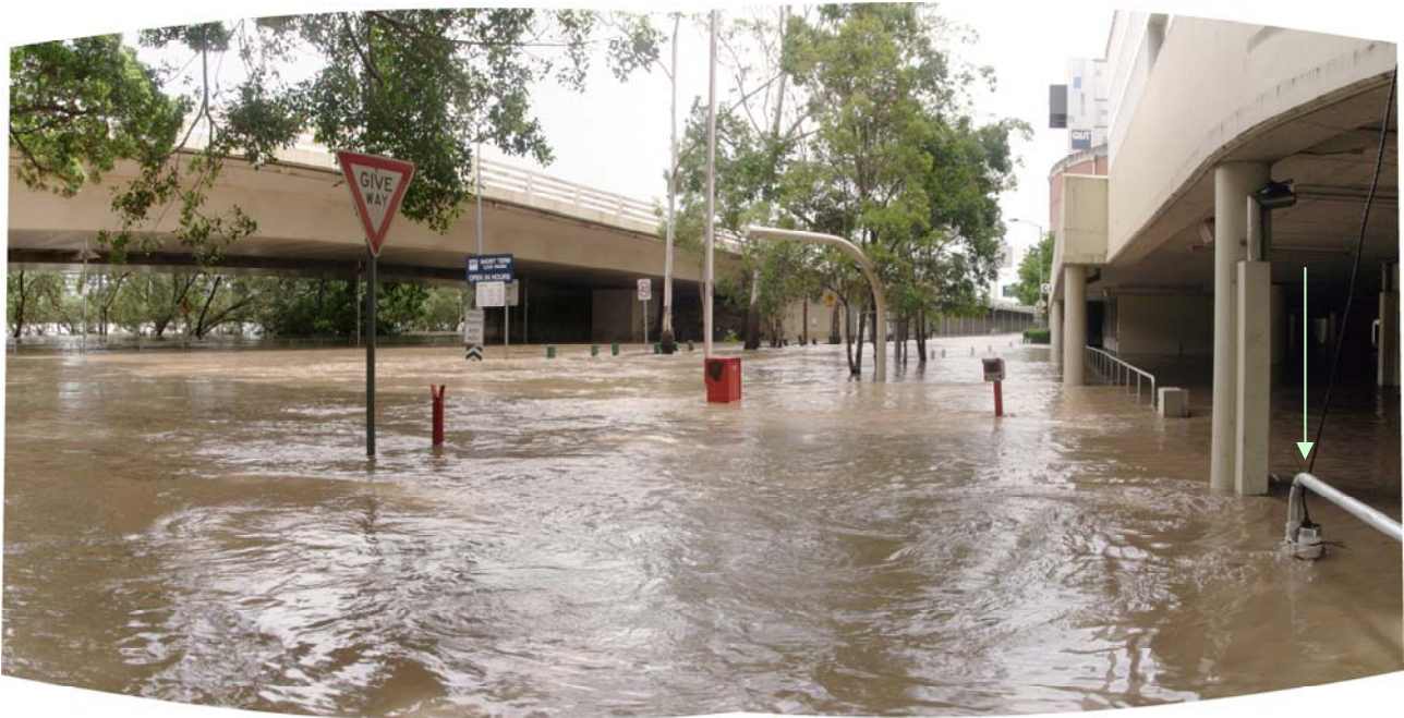
Gardens Point Road on Thursday 13 January 2011 at 11:39 - Note the ADV system on the far right
