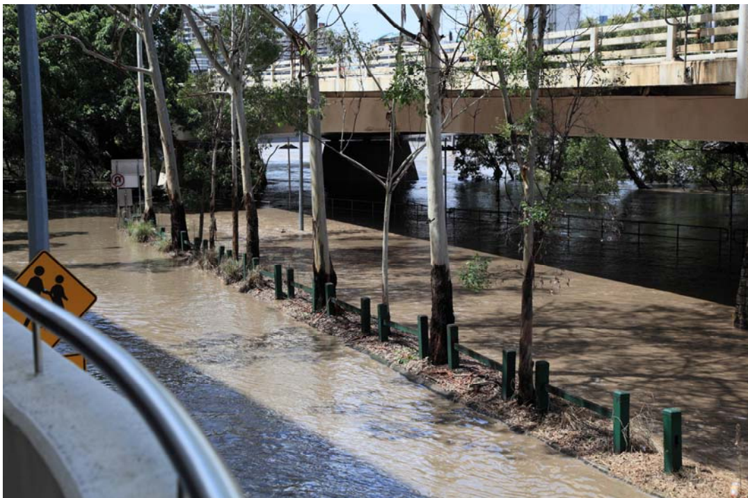
Fig. A-5 - Gardens Point Road looking SE (downstream) from C Block on Wednesday 12 Jan. 2011 at 10:08 (Photograph QUT Facilities Management) - Canon™ 5D Mk II with Canon™ EF24-105mm F4L IS USM lens - Flow direction from bottom right to background; the main channel of
