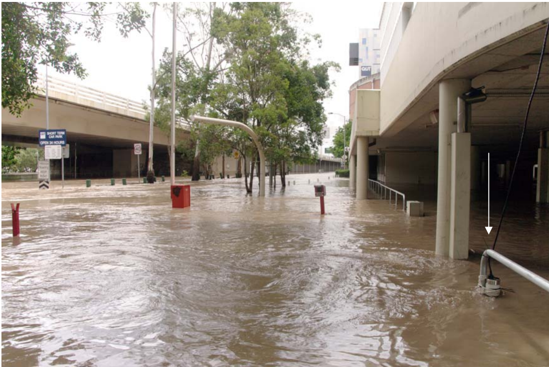
(A) Submerged ADV system in operation (arrow)
