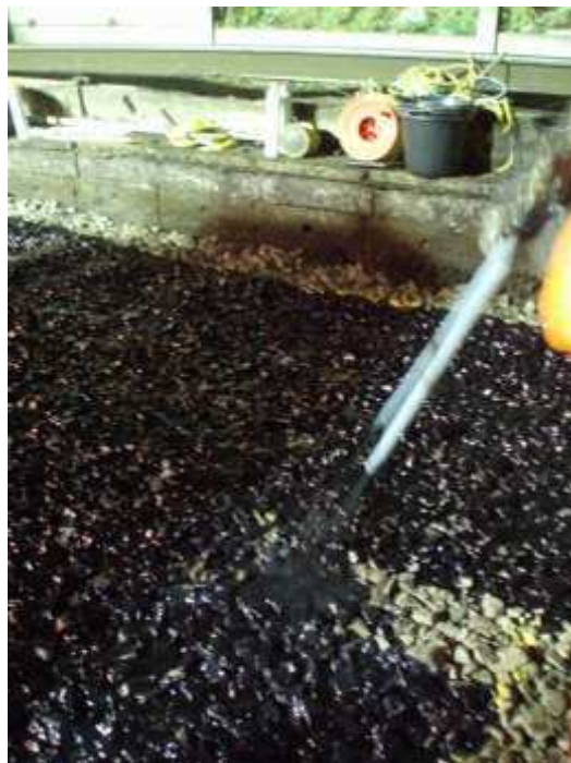
Figure 10: Pouring of the polymer at the site
