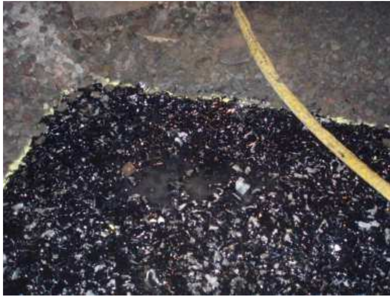
Figure 11: Water rising up through the GeoComposite layer during polymer pouring
