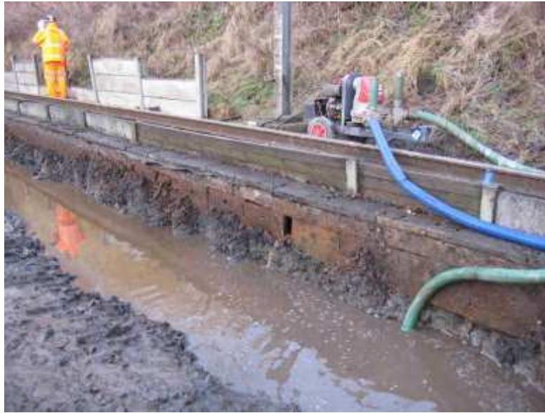
Figure 9: Application of pumps to try and drain water during installation
