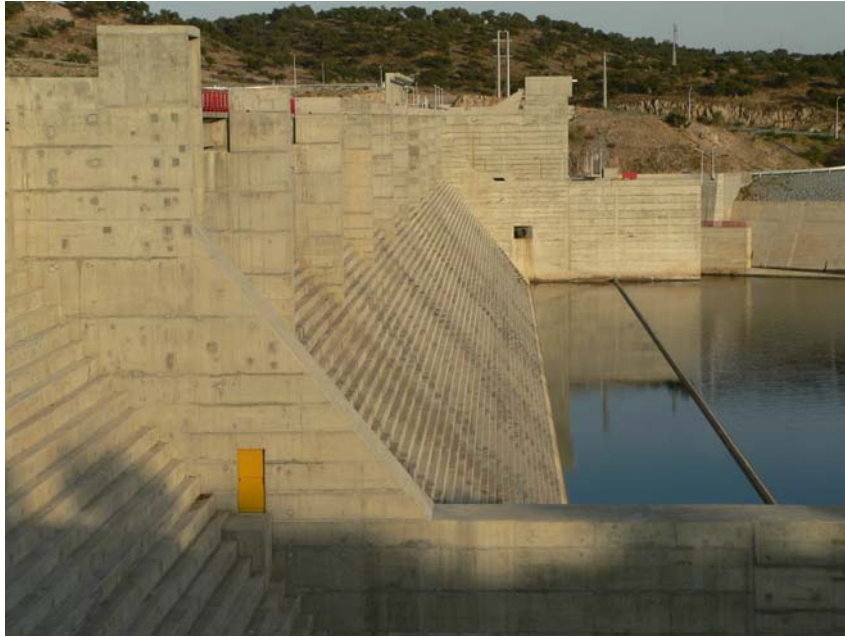
(A) Stepped spillway on 4 September 2006
