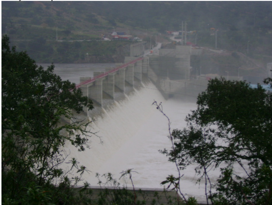
(B) Skimming flow on 16 January 2010 with a discharge 1,000 \text{ m}^3/\text{s} , \text{Re} = 1.3 \times 10^7 (Courtesy of Professor Jorge MATOS)
