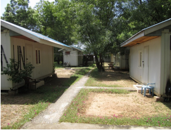
Containers with A/C and hot water, UN accommodation, Bor.
