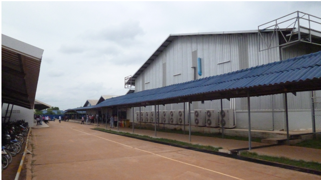
Figure 9: Workers Outside Savannakhet Factory. 18
