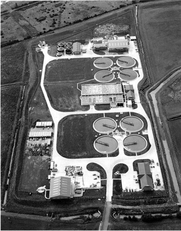
Figure 5.6 Typical sewage treatment works the circular vessels are settling tanks, the rectangular structures in the centre are aeration tanks. At the rear of the site are sludge digesters. Spent sludge is spread at the far end.
