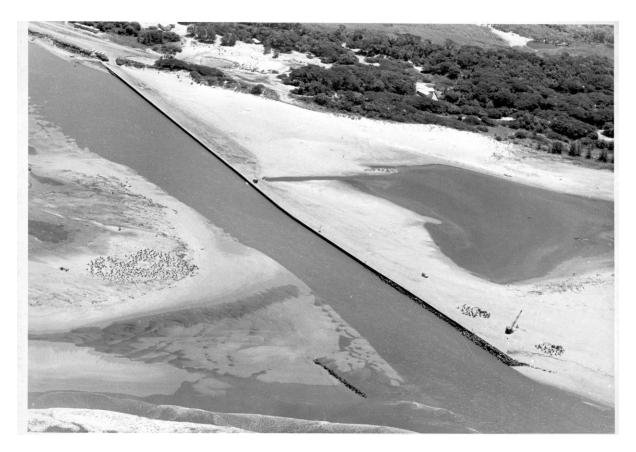
Fig. 7. Aerial photograph of the St Lucia mouth showing the partially constructed groynes designed to stabilize the north and south banks of the estuary. In the mid-left of the picture is a stockpile of dolosse used to reinforce the groynes adjacent to the sea (Photo: R.H. Taylor, 1976).
