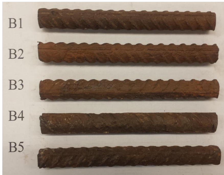
Figure 7.1 Typical picture of the corroded parts of the bars of all tested beams
