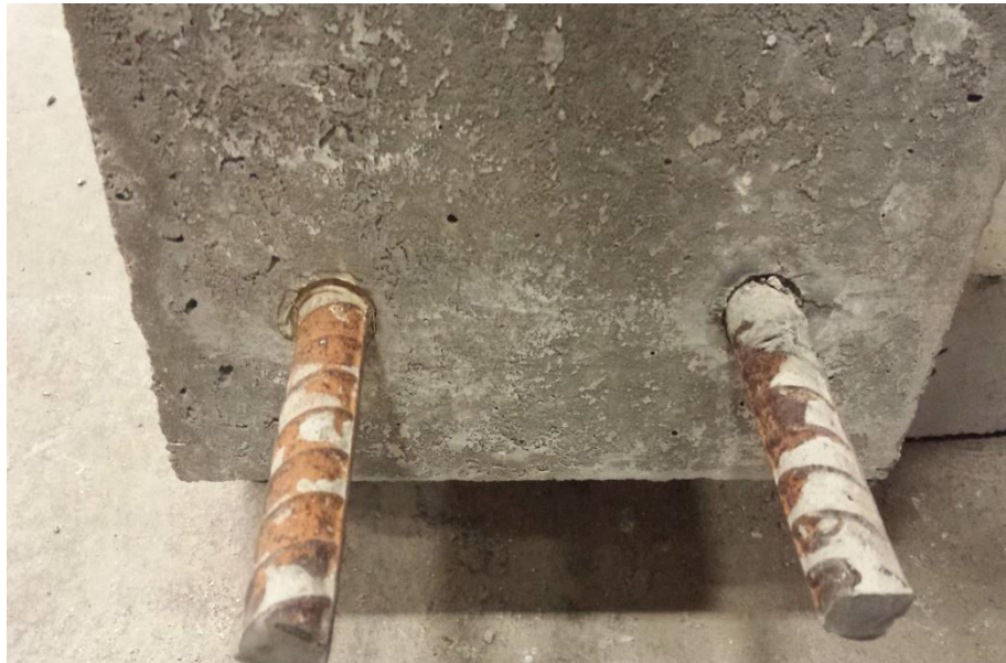
Figure 7.7 Bar slippage in B9 after failure
