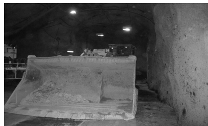
Figure 2: The underground environment
