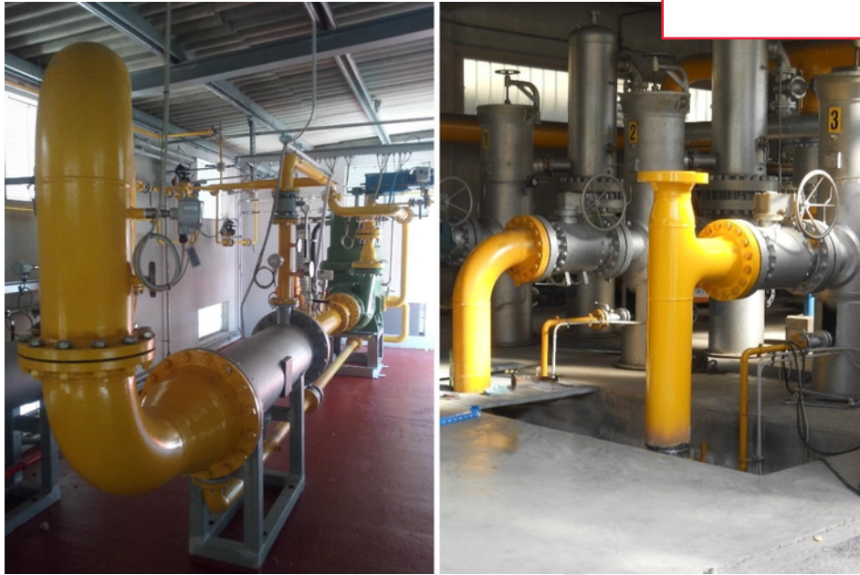
Fig. 1. GE1 demonstrator (left: turboexpander; right: throttling valves).
