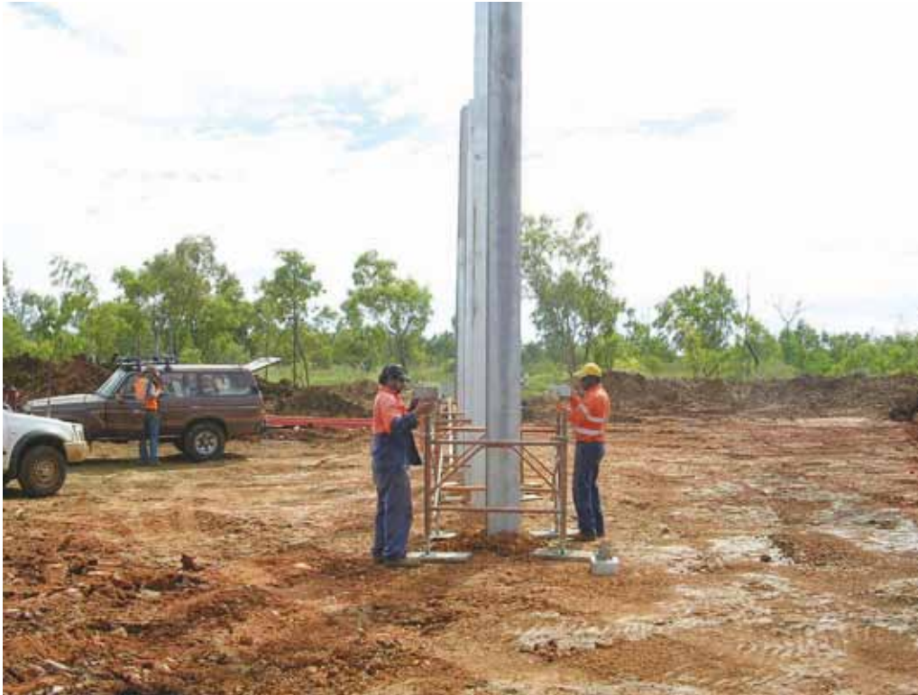
Figure 8: Barkly Highway upgrade, installation of bridge footings and piers
