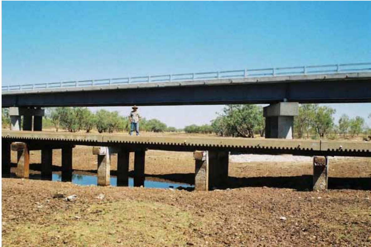
Figure 6: The old Georgina River bridge in front of the new bridge
