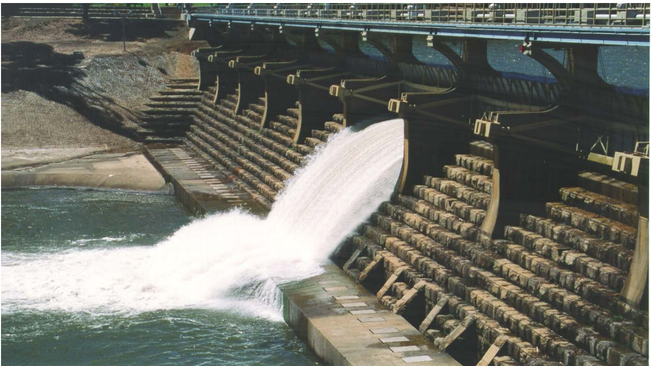
Fig. 2 - Goulburn weir (Australia) on 30 Jan. 2000 (Photograph H. CHANSON) - Flow rate: Q = 5.2 \text{ m}^3/\text{s} , Step height: h = 0.5 \text{ m} - Gravity overflow weir completed in 1891 on the Goulburn River (Victoria)
