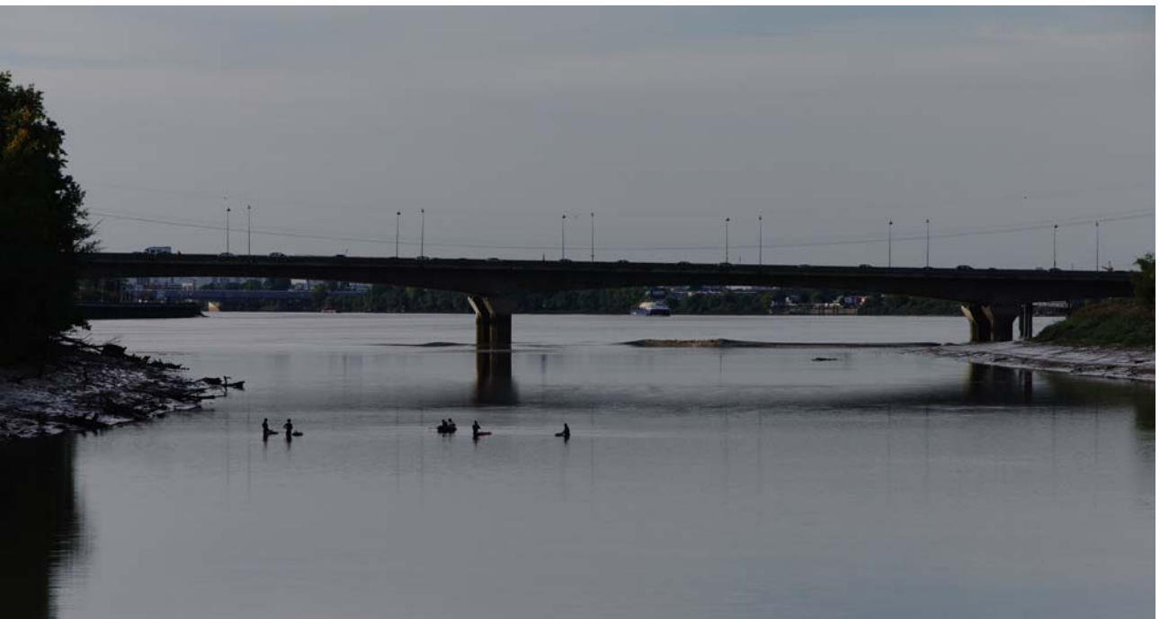
(B) At 18:54:50 - Note the Airbus barge in the background travelling upstream to Langon behind the tidal bore, and the surfers in the foreground standing next to their surf boards
