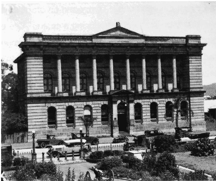
Figure 2: former state library William Street 1931 (JOL 185381p)
