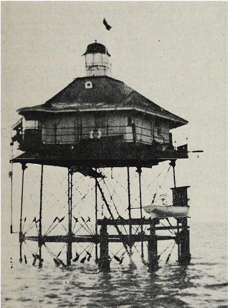
The Old Pile Light 1885.
