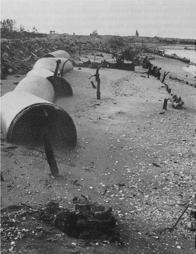
The remains of the Lucinda in mid February 1993, viewed from the stern looking towards the bow along the length of the ship. The large concrete pipes, dumped there as landfill, lie parallel to and inboard of the port side which is actually covered by the rocks of the temporary causeway. The exposed starboard ribs, projecting for less than half a metre above the sand, can be seen from the mid right towards the top centre of the photo. A subsidiary line of ribs to the right of these ribs belongs to the port side remains of the Moreton. Within the Lucinda proper, the rudder post is at the bottom of the photo, while the remains of certain pillars and a transverse bulkhead are to be noted within the ship's outline. The objects on the skyline are heavy earth moving units. G. Martin and D. Martin
