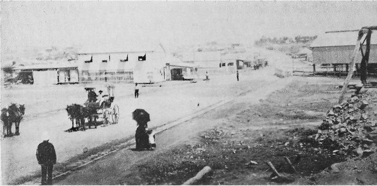
Lower Gill Street and Millchester Road near the Railway Station, Charters Towers. (R.H.S.Q. Collection)
